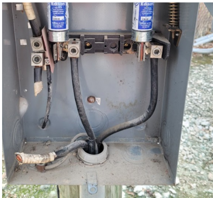
Left: Successful cuts and theft of wire in equipment cabinet. Top right: Cuts to wires on utility pole in conduit. Bottom right: Cuts to wires on utility pole in cabinet.
